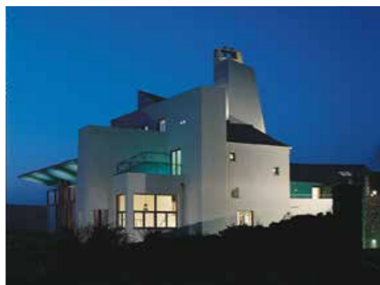
Baggly House - Devon, UK DRYVIT PROJECTS
